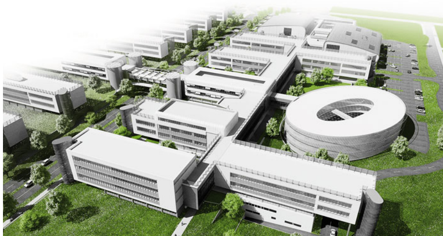
CEITEC laboratories in Brno – Bohunice University campus
